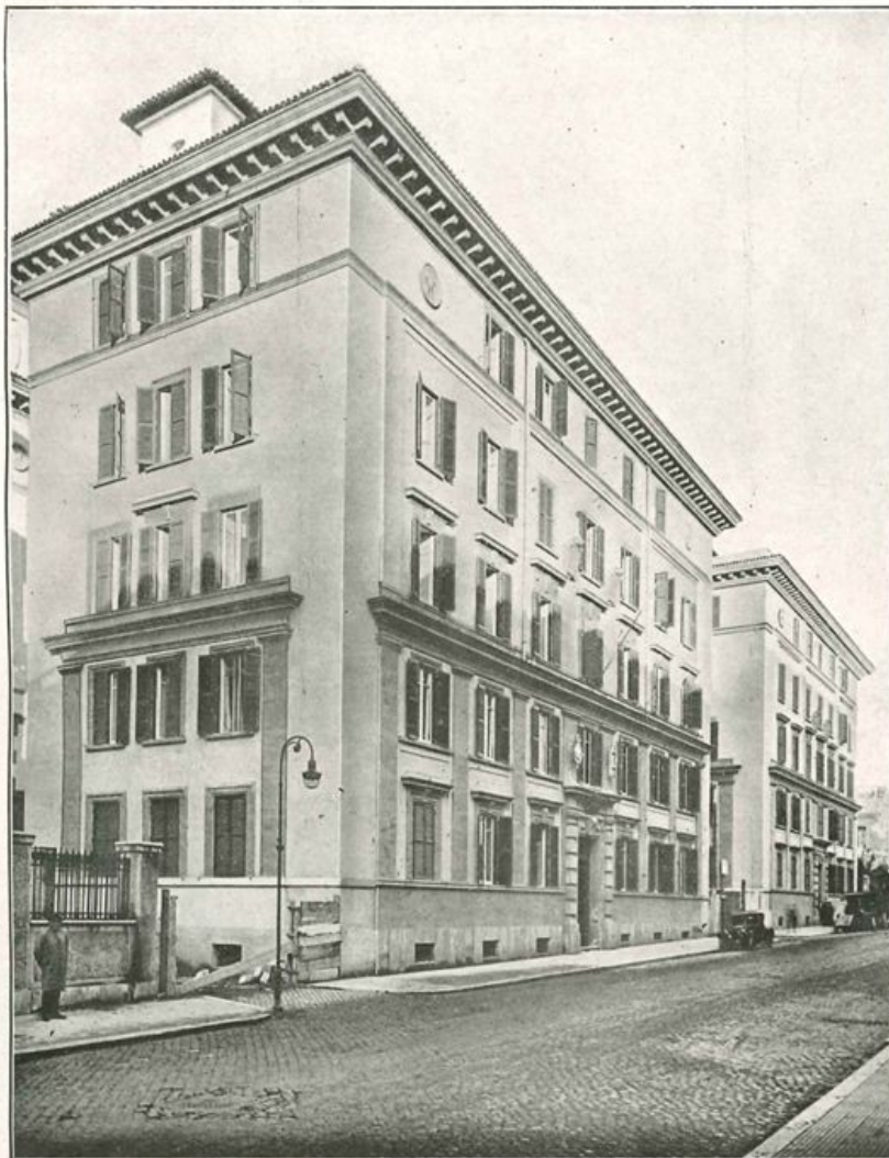
ROMA - PALAZZINE IN VIA SAN QUINTINO (5 PALAZ- ZINE)
